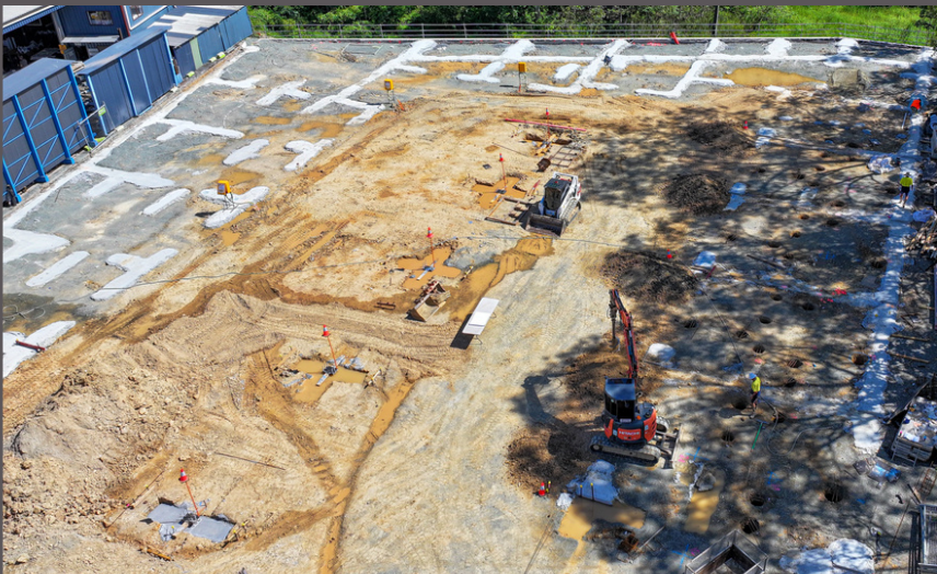
STRUCTURAL FOOTINGS INSTALLED
