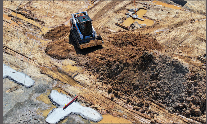
SITE EARTHWORKS COMPLETED
