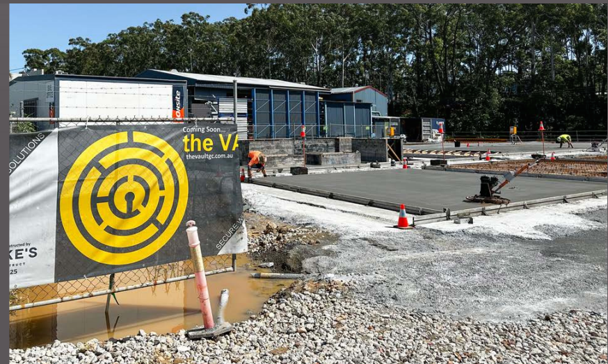
FRAMING & POURING OF CONCRETE PANELS
